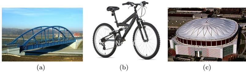
**Fig. 1** Structures are typically composed by interconnected rigid bodies and they can have different types of mobility. (a) A fixed bridge is an example of rigid structure. (b) The shock absorbers of a bike are passive mobile structures (c) Retractable roofs are active structures.
